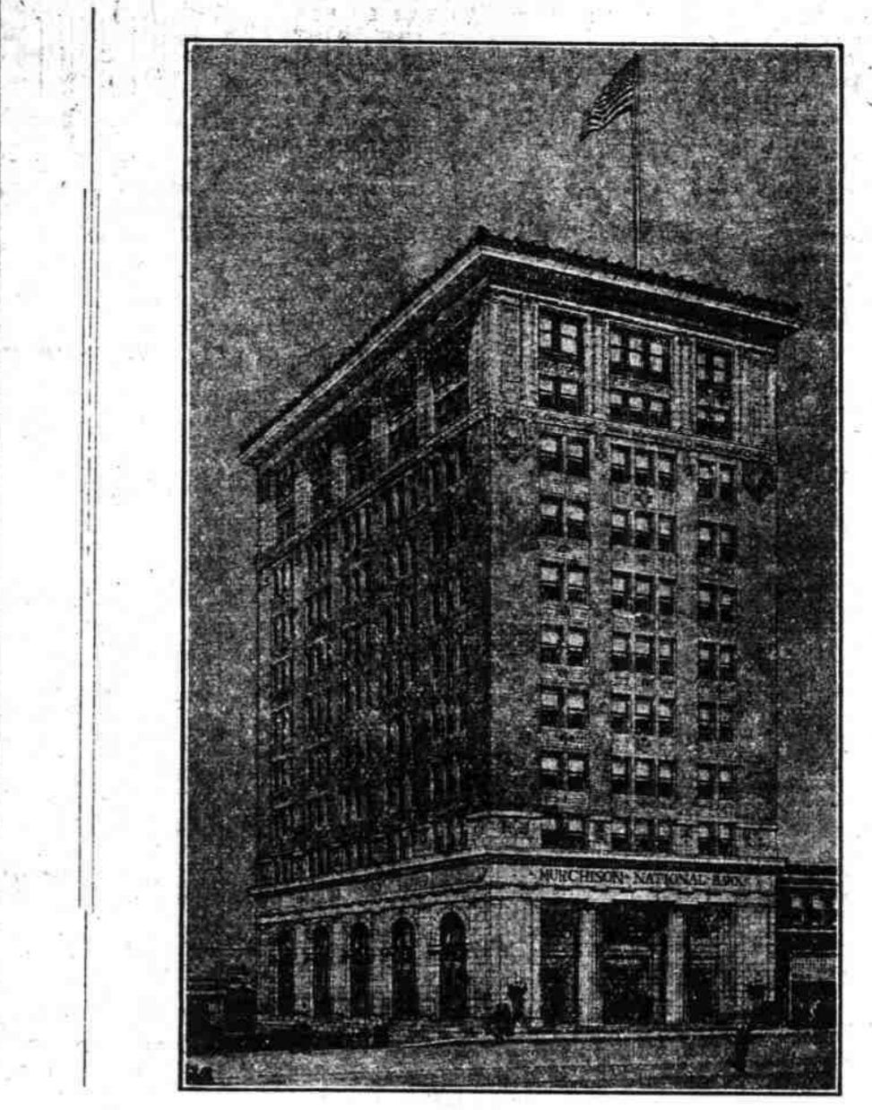
To be erected for Murchison National Bank; 65x106 feet; 10 stories; fireproof construction; slag roof; steel heating; 3 electric elevators; cost $2,750,000; architect, Kenneth M. Murchison, New York; construction bids opened soon.
