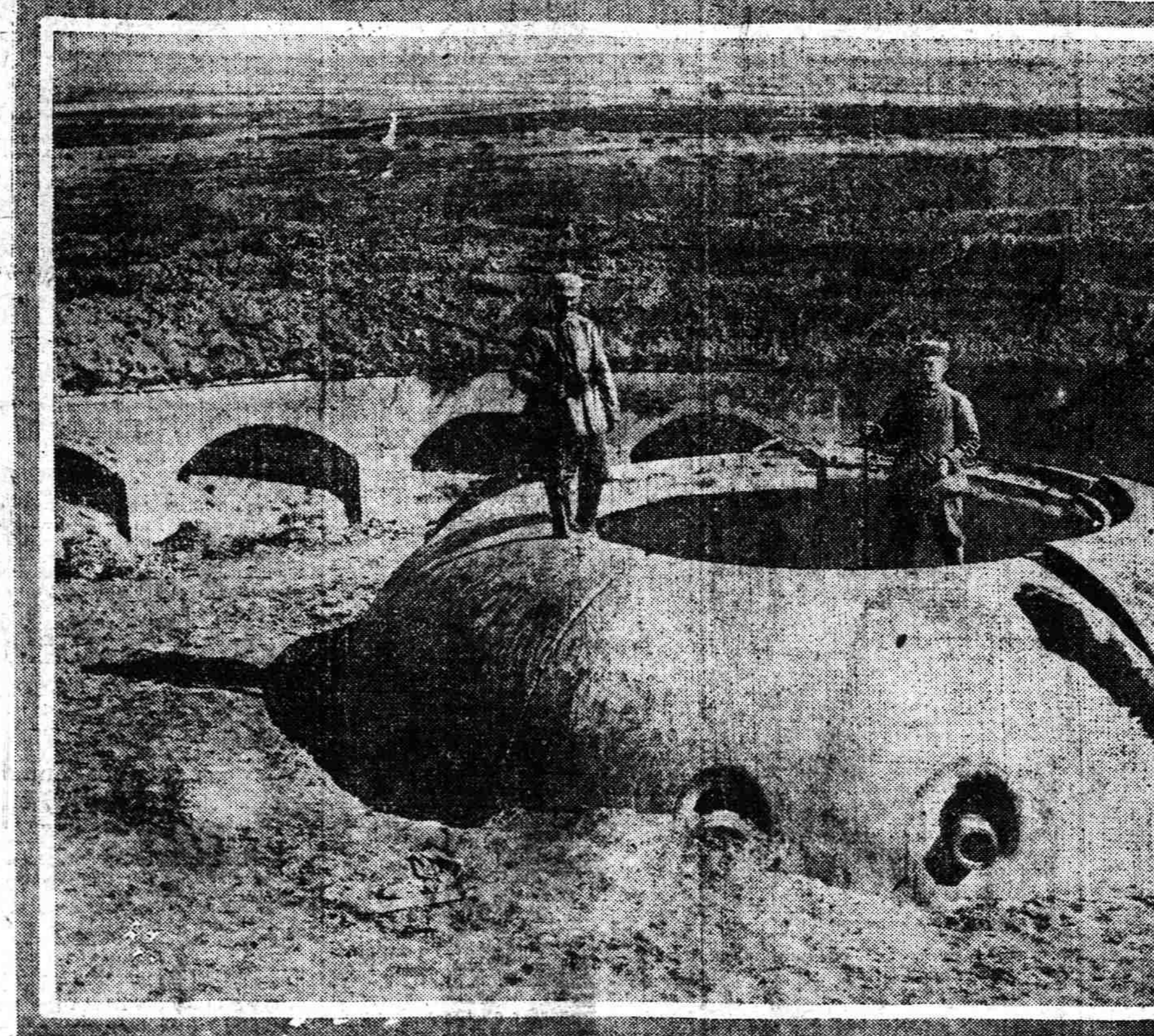
The rent in this thick steel enclosure at the great French fortification at Longwy, near the German border, shows the enormous power of the German 16-inch gun. The fort was taken by the army under Crown Prince Frederick, and was the second of the great French fortresses to succumb to the new German gun. After the Germans had taken Liege and Namur with the aid of this gun they moved on to Mauberge, and that city did not last long.
