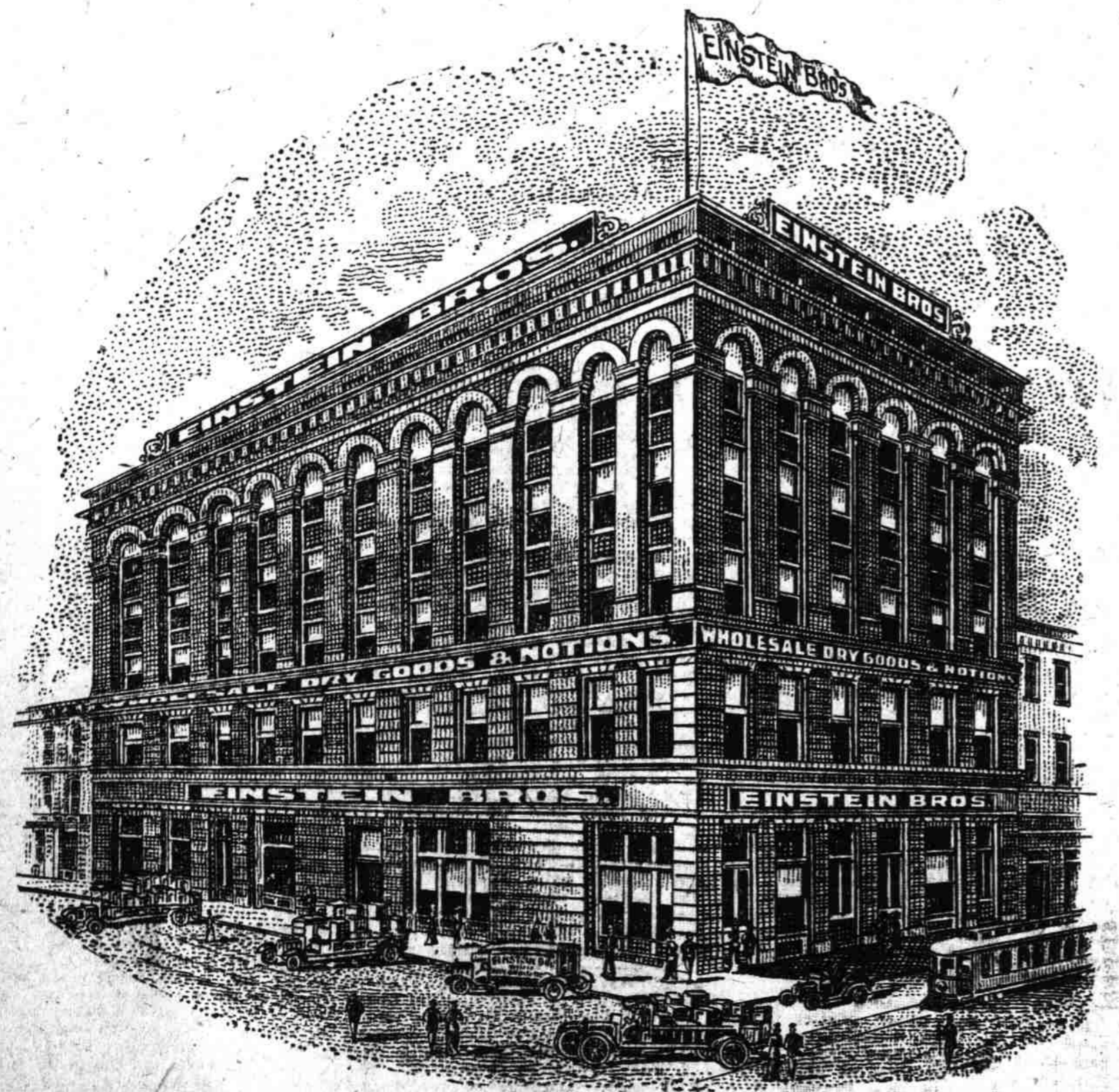
EINSTEIN BUILDING, FRONT AND GRACE STREETS, PURCHASED BY EFIRD BROS.
