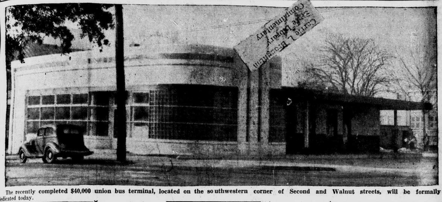
The recently completed $40,000 union bus terminal, located on the southwestern corner of Second and Walnut streets, will be formally dedicated today.
