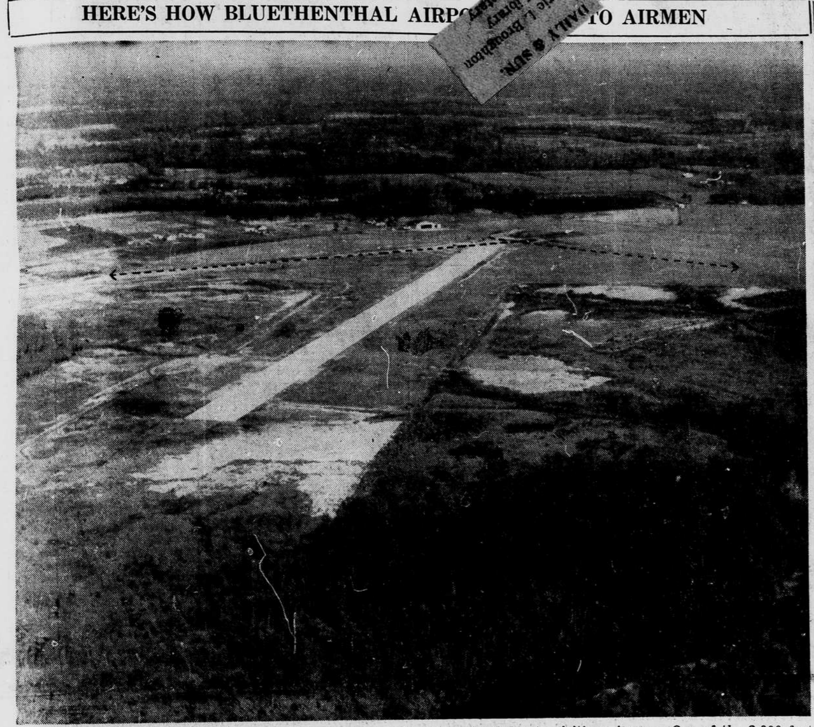
Here is Bluethenthal airport, located on the Gordon road, as it looks today to visiting airmen. One of the 3,000 feet long, 100-foot wide runways has been covered with a rock base and the dotted lines show where the other two runways are to be constructed.
