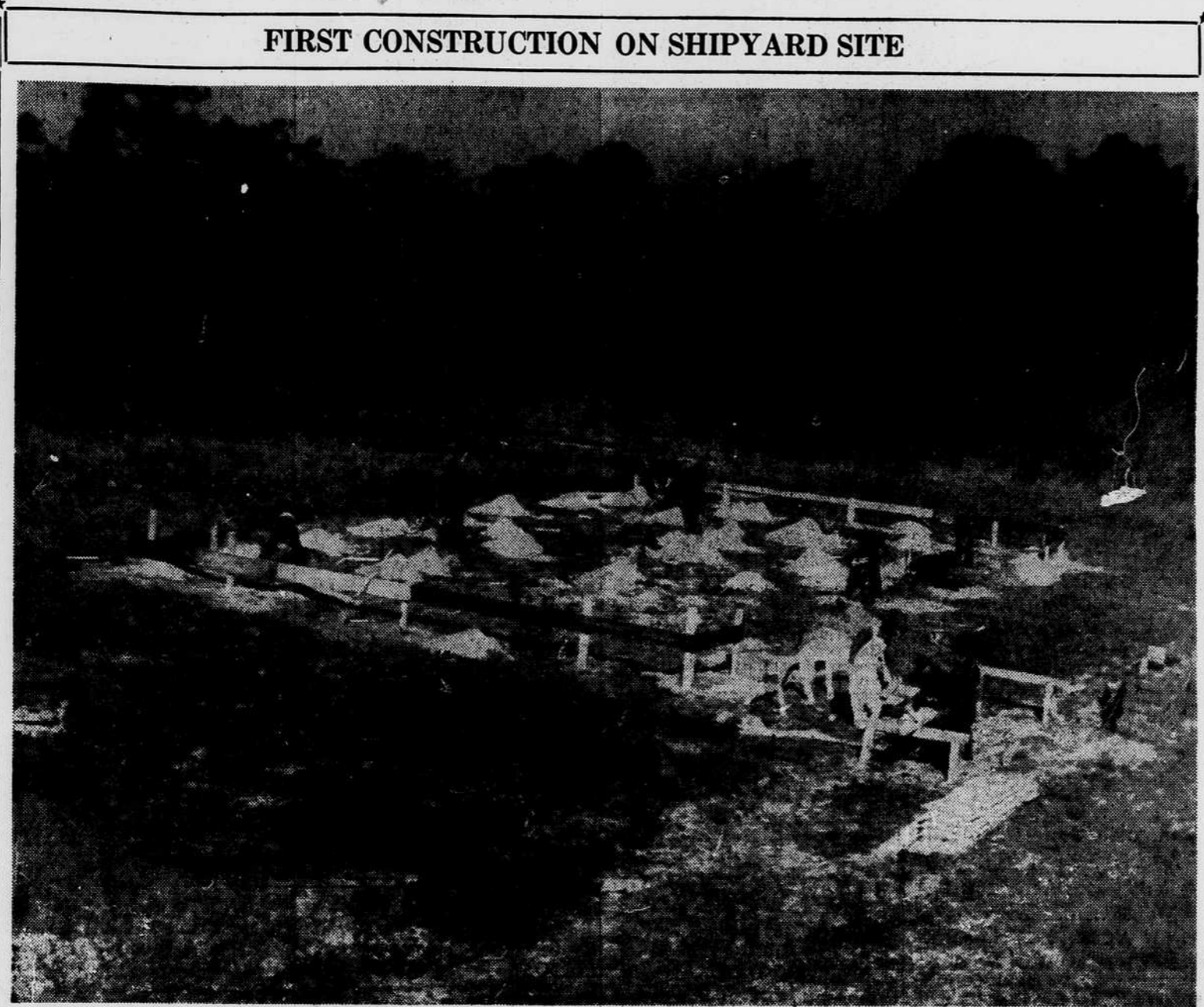
Shown above is the first construction at the Wilmington shipyards of the North Carolina Shipbuilding company being erected at Sunset Park on a 70-acre site. This building will stand at the southeast corner of the tract and will be used as a temporary office by Loftis, Underwood and Orrell, associated contractors.
