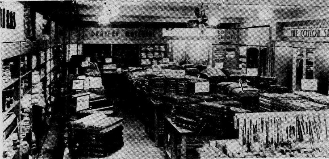
NEW ADDITION—This is a view of the new second floor addition to the J. C. Penney Co. Among departments arranged on this floor are the draperies, infant wear, domestics, piece goods, foundation wear and cotton shop.
