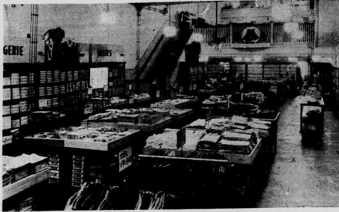
STORE ENLARGEMENT—Photo shows partial view of first floor of the J. C. Penney Co. The rear of the store contains the new department for boys' wear and enlarged shoe department.
