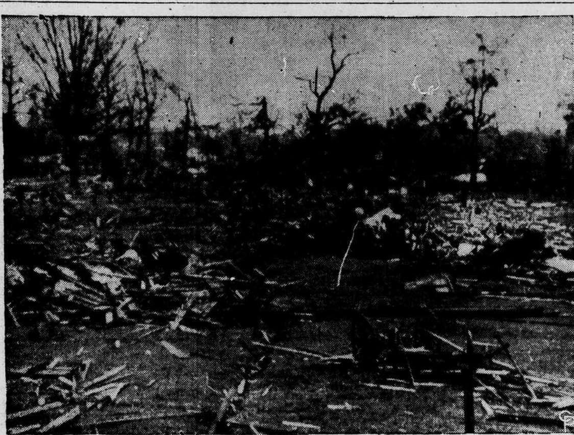
DEATH BLOWS THROUGH ARKANSAS—13 KILLED Kindling wood is all that was left when a tornado tore through Hamburg, Ark., destroying 30 homes and killing 13 persons. Shown above are some of the homes blasted by big wind, with not even one wall standing.—Central Press Photograph
