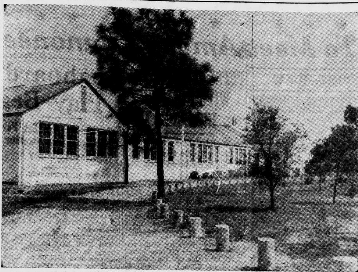
The newly completed right wing addition to the Carolina Beach school is expected to accommodate the heavy influx of children during the coming year. The addition, built by the Federal Works Agency as a war public works project, was completed recently. (Federal Works Agency photo by Zerwick).
