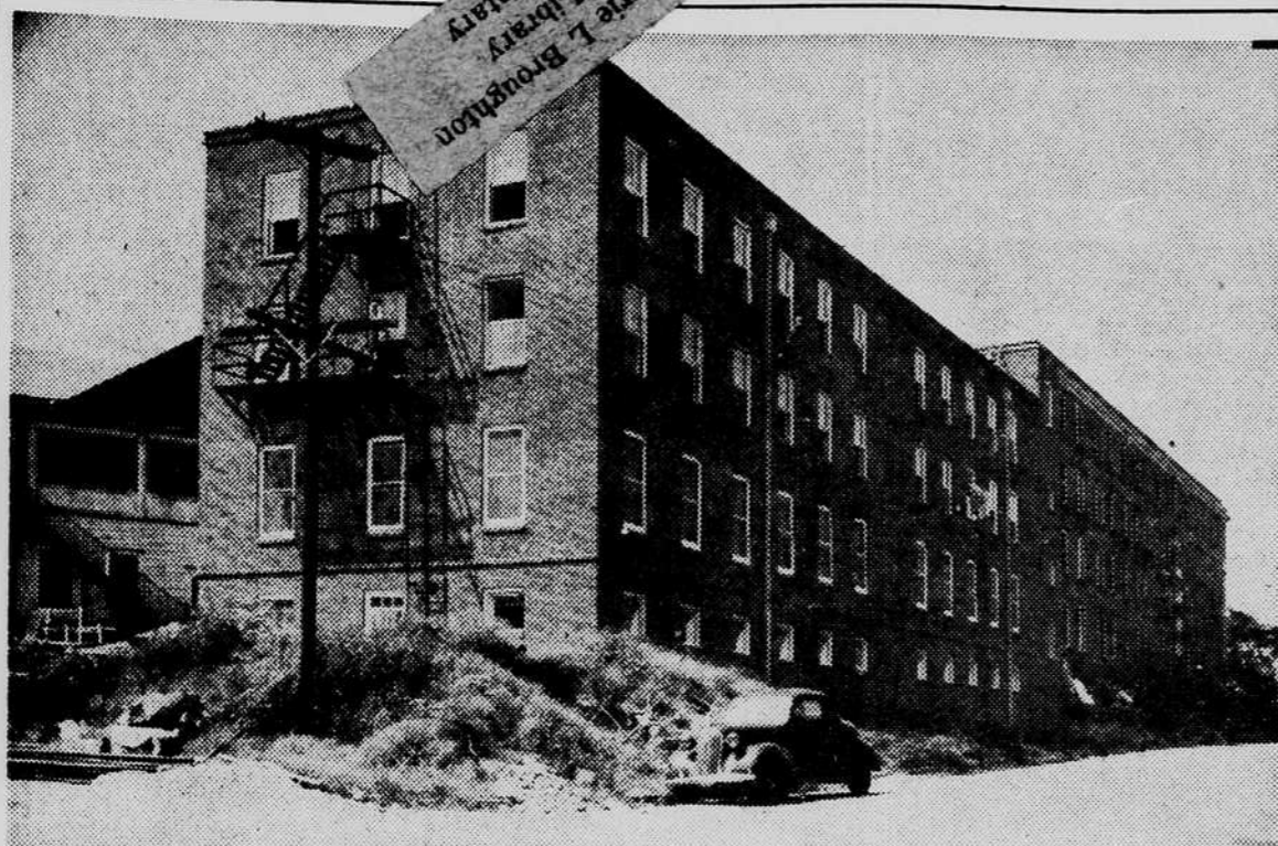
The four story addition to the nurses' home at James Walker Memorial hospital is now complete and has been turned over to the board of managers by the Federal Works Agency. The structure will provide living quarters for 70 nurses. C. F. Churchill, FWA engineer, declared. Equipment for the interior has not been received but temporary provisions for occupancy have been made.
