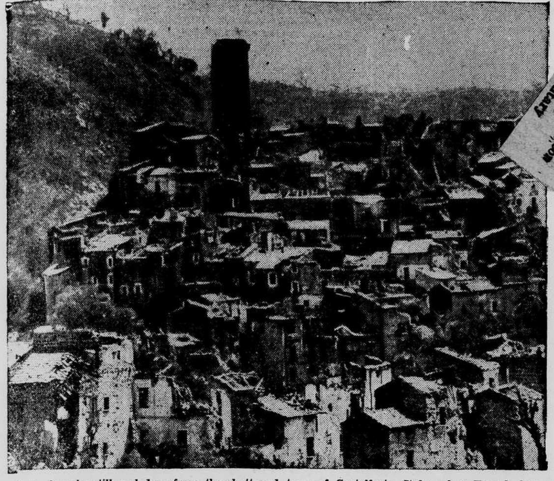
Wisp of smoke still curled up from the shattered town of Castelforte, Italy, when French forces entered on the heels of the retreating Nazis. Before the town was captured it was a link in the Gustav Line. The effects of the terrific Allied shelling are clearly discernible. This is a U. S. Signal Corps photo. (International)
