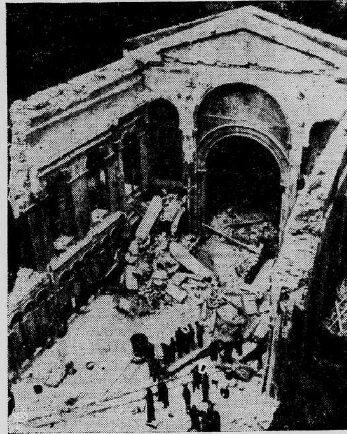
Salvage workers clear the wreckage from the famous Guards Chapel, between Buckingham Palace and the Parliament Buildings in London, after it was struck by a Nazi robot bomb. The 106-year-old chapel was hit during services and casualties are reported to be heavy. Note that only one end of the chapel is left standing.
