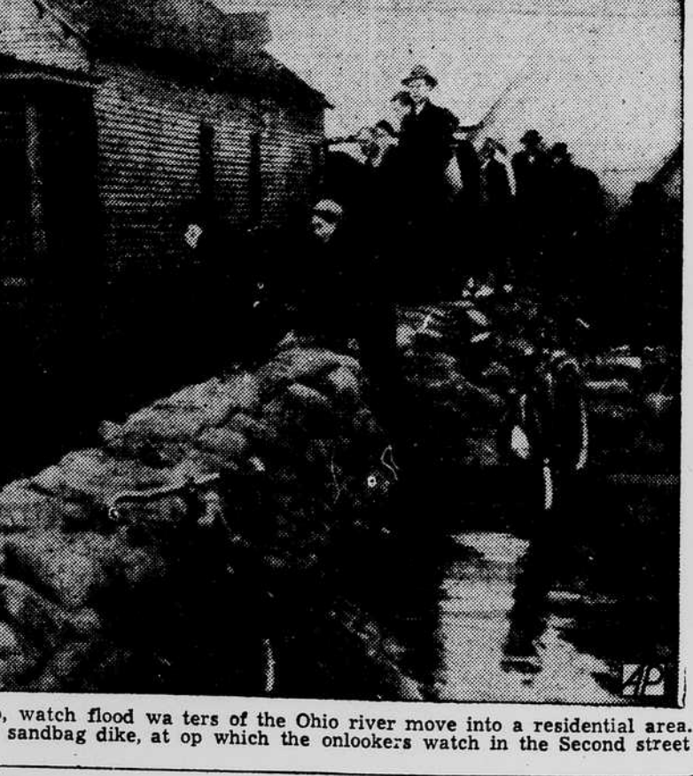
Residents of Portsmouth, Ohio, watch flood waters of the Ohio river move into a residential area. Soldiers and volunteers threw up a sandbag dike, at top which the onlookers watch in the Second street area. (AP Wirephoto)
