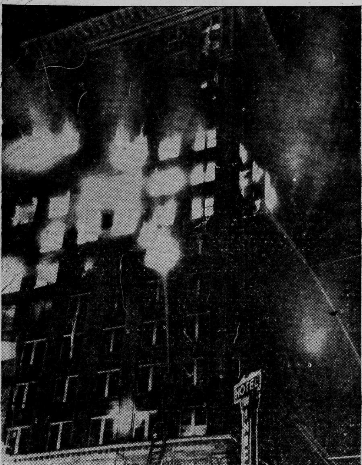
TAKEN AT THE HEIGHT OF THE FIRE in the Wincoff Hotel in Atlanta, Ga., this photo shows flames roaring through the upper floors. At least 120 persons, according to early reports, died in the conflagration. The 350-room structure is located on famous Peachtree Street. (International Soundphoto).
