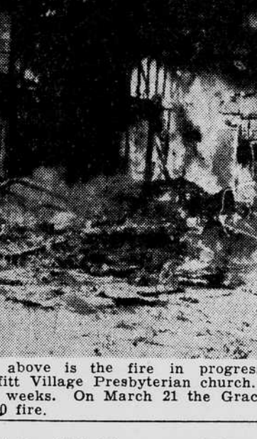
CHURCH DESTROYED—Pictured above is the fire in progress yesterday which did an estimated $15,000 damage to the Maffitt Village Presbyterian church. This was the second church fire in this area during the past three weeks. On March 21 the Grace Street Methodist church in Wilmington was destroyed in a $200,000 fire.
