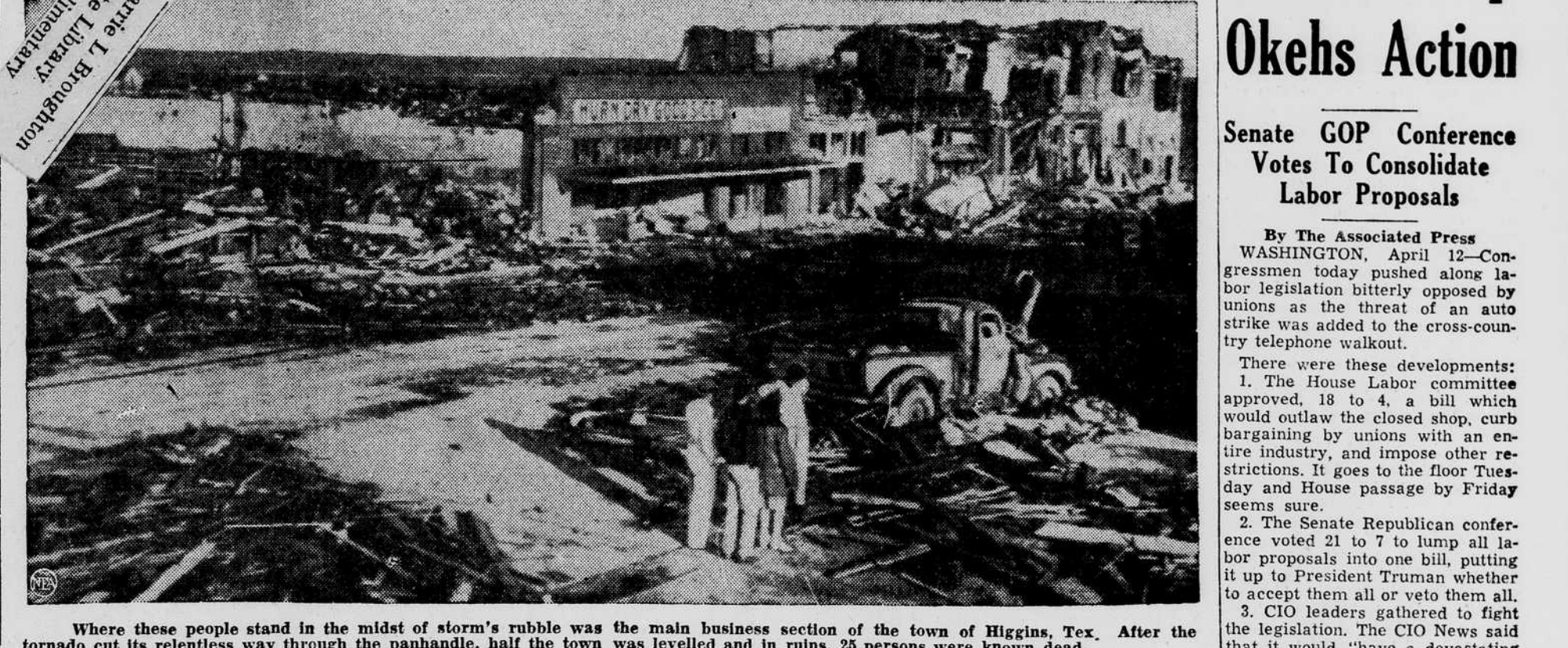
Where these people stand in the midst of storm's rubble was the main business section of the town of Higgins, Tex. After the tornado cut its relentless way through the panhandle, half the town was leveled and in ruins, 25 persons were known dead.
