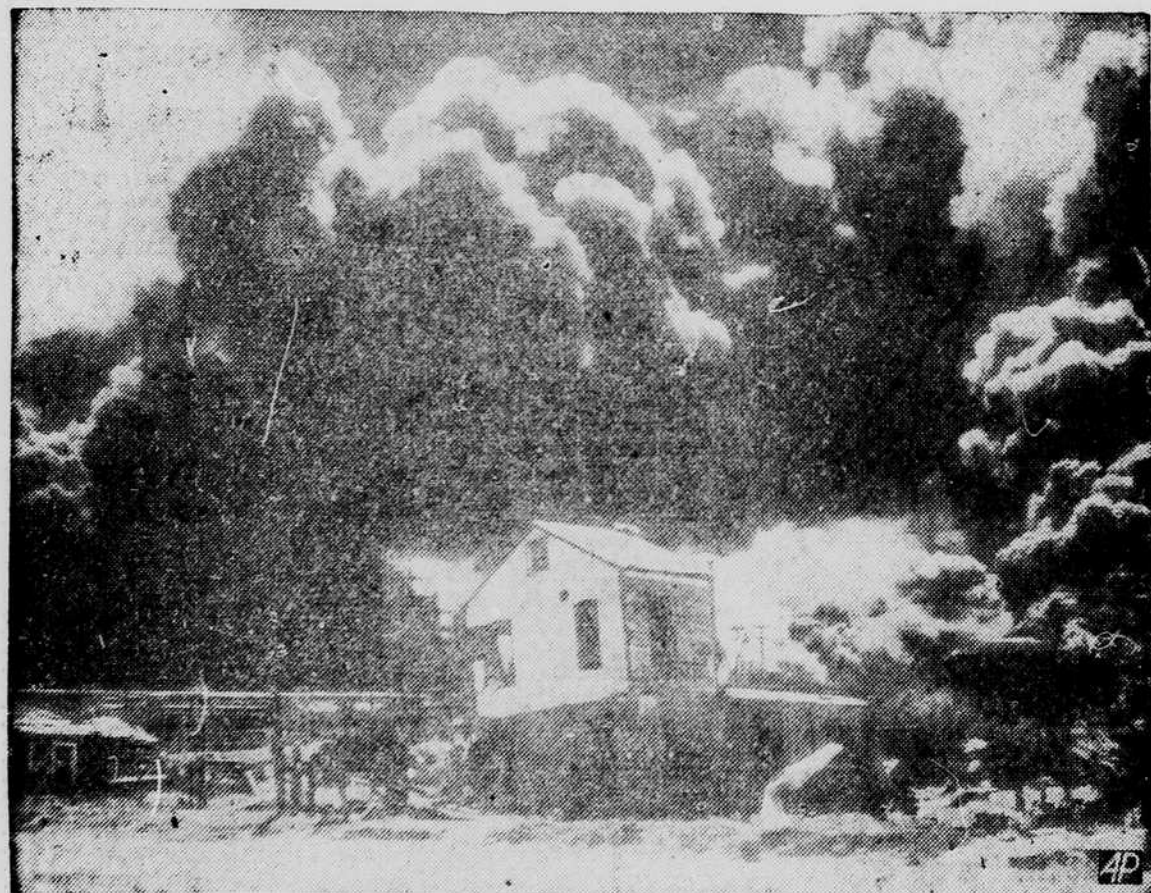
TEXAS CITY PLANT ENGULFED IN SMOKE—AN IMPENETRABLE CLOUD of smoke engulfs the plant on the Monsanto Chemical Company in Texas City, Tex., following a series of explosions and a fire which virtually razed this city of 15,000 persons. More than 1000 were believed dead, in the worst explosion disaster in Gulf Coast history. Wire reports indicated that several thousands of town-folk had been attracted to the waterfront by a fire aboard a French ship, which was taking on nitrates. Suddenly the ship blew up, taking an immediate toll of some 500 lives, with thousands injured. A second explosion and fire then rocked the chemical plant, bringing more casualties.—(International Soundphoto).
