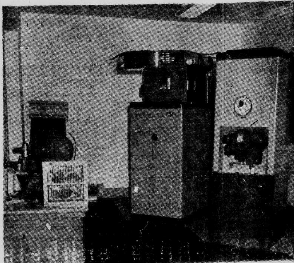
The Hanover Iron Works showroom at 112 North Water Street showing the Lennox Aire-Flo basement type oil-fired winter air conditioning unit. The duct work on top of furnace, with streamers at air outlets, shows principle on which rotary blowers in furnace casing operates. The other model is the smaller Lennox utility model which operates on the same principle.
