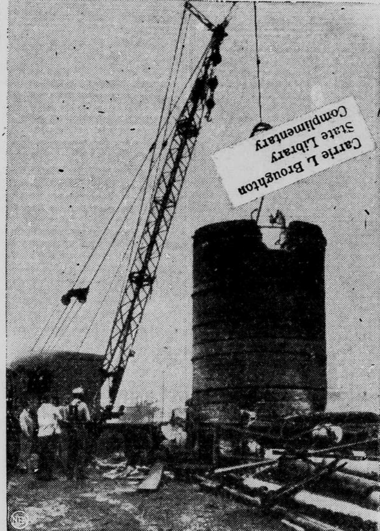
Complimentary State Library Carte L. Broughton FOUR SOCIALLY PROMINENT MASSACHUSETTS residents died when their chartered plane crashed into this 40-foot high brick furnace at Everett, Mass. Here a crane lifts the burned remains of the fuselage from inside the cauldron. Dead were identified as Thomas Mandell, 55, Boston broker, his daughters, Ann, 22, and Harriet, 19, and John Nelson Borland Pell, 32, pilot.
