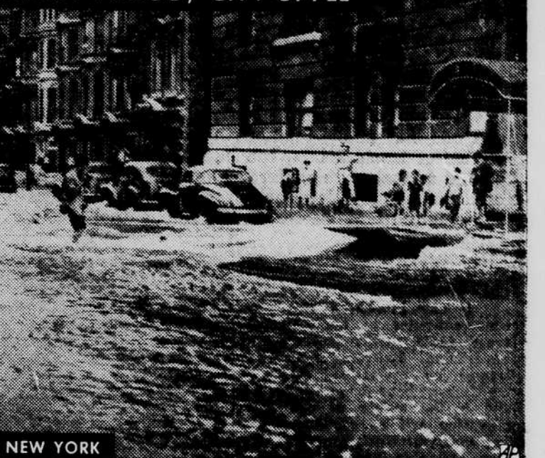
METROPOLITAN streets were flooded three feet deep over a four-block area when 48-inch water main burst beneath the pavement. Though no fatalities were reported, damage was set at several thousands of dollars.
