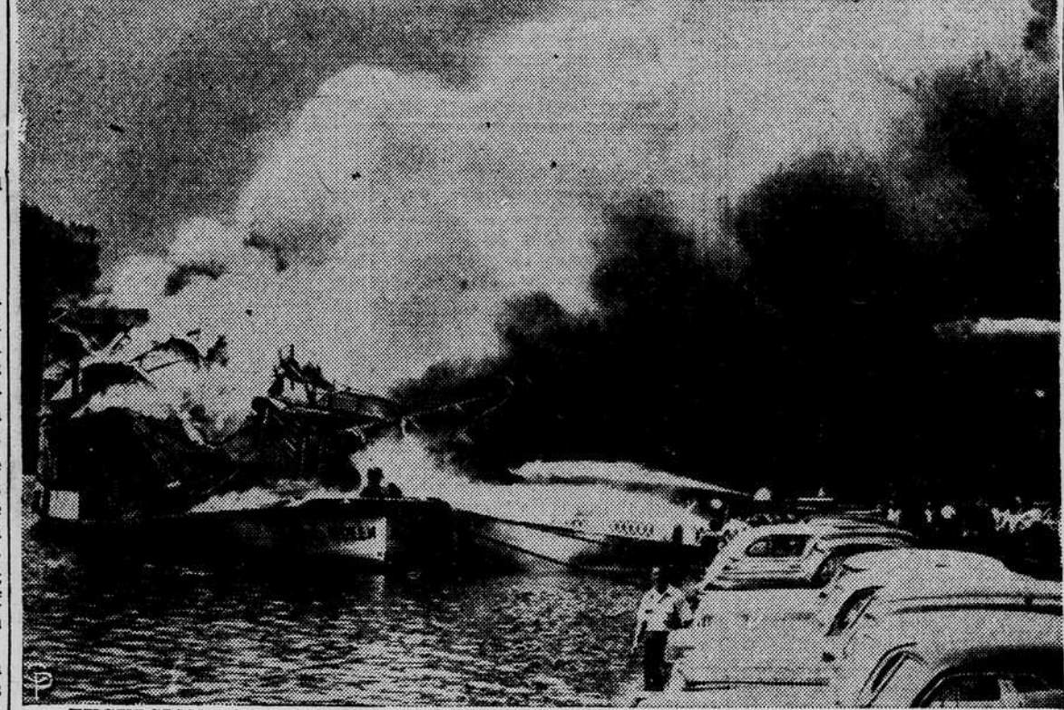
EXCURSION BOAT AFIRE after death blast. Hoses are played on the blazing river excursion boat "Island Queen" following the blast which occurred as the craft was tied to its dock in the Ohio River at Pittsburgh. Though the boat normally carries a crew of 96, police reported that fortunately many were ashore at the time of the explosion. Twelve persons were said to have lost their lives. (International Soundphoto)
