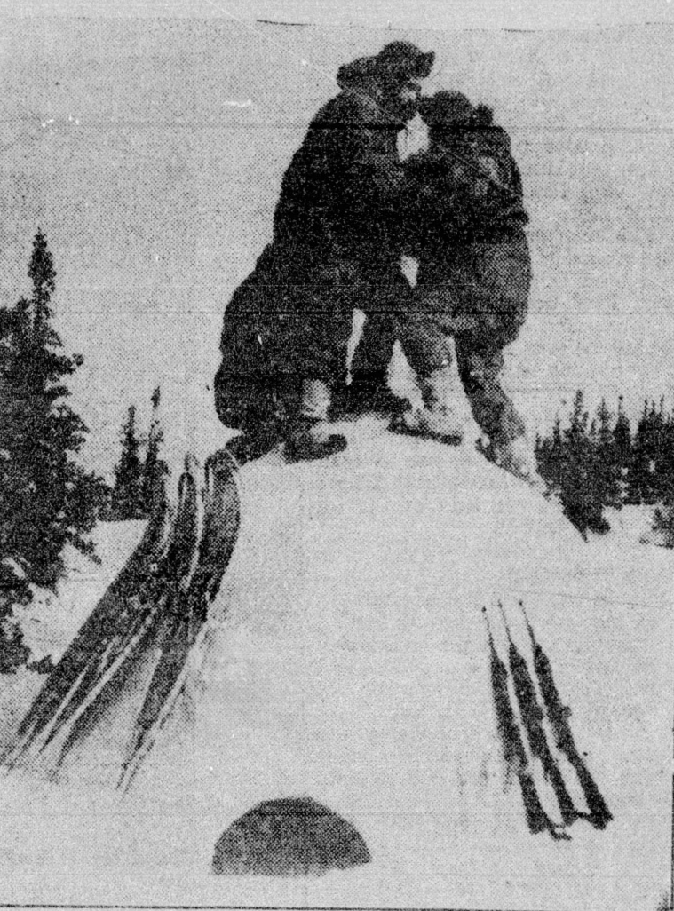
TESTING THE ROOF OF AN IGLOO—These soldiers of the U. S. Arctic Infantry patrol have completed a snow hut on the shores away up north and are making sure that the dome will withstand more than 500 pounds weight. These huts provide shelter for troops for many weeks.
