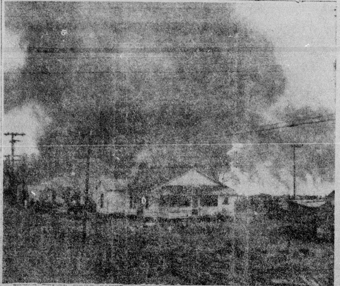
AT FUQUAY-VARINA BLAZE — The above picture was taken as firemen battled to control flames which caused more than $128,000 damage Monday as they destroyed the New Deal Tobacco Warehouse and gutted four nearby homes shown in the foreground. Firemen from Angier, Apex, Dunn, Fort Bragg and Raleigh joined in fighting the fire. Damage to the four homes was estimated at $1000. Owners of two of them, Mrs. Elsie Balfour and J. D. Elliott, lost all of their belongings. Residents of the other dwellings, however, were able to save most of their clothing and furniture. The explosion of several oil drums in the rear of the warehouse aided in the spread of the blaze. — Photo courtesy of The Raleigh Times.
