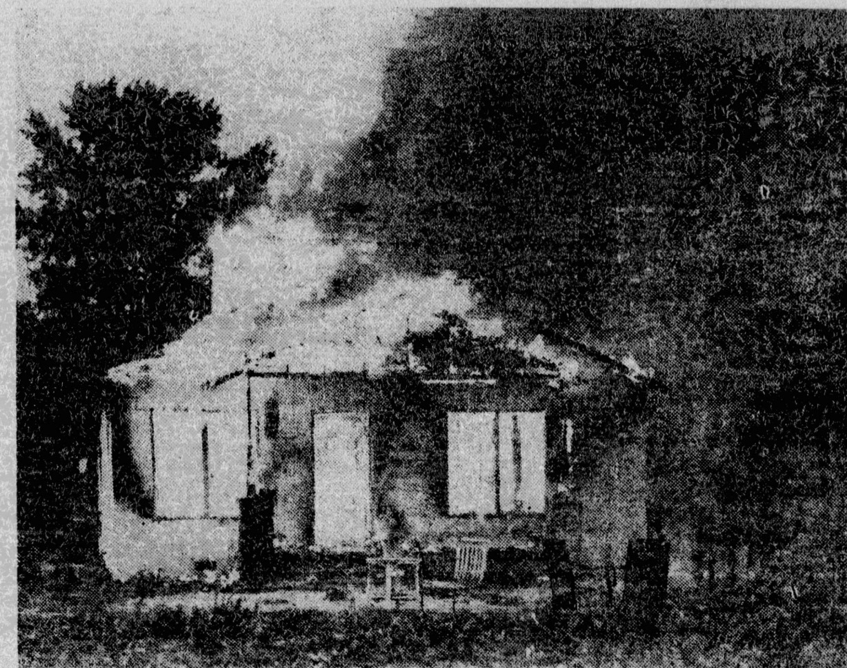
COMPLETELY DESTROYED— Fire completely destroyed the residence of Mr. and Mrs. Elbert Lee of Smithfield. Only the two chairs and porch furniture shown in front of the burning structure were saved. Lee is being held on an arson charge. Photo by Herman D. Lawson. Courtesy of News and Observer.
