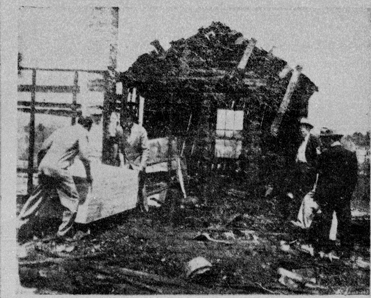
Above is all that remains of a house in which the body of Boise Pearson, 33, was found early Friday morning. The two men in the left hand corner are undertakers who are bringing out the body of Pearson, who was a roomer in the house. With back to camera are Marshall Edwards and L. C. Fritchett, constable of Cross Creek Township and J. J. Township.
