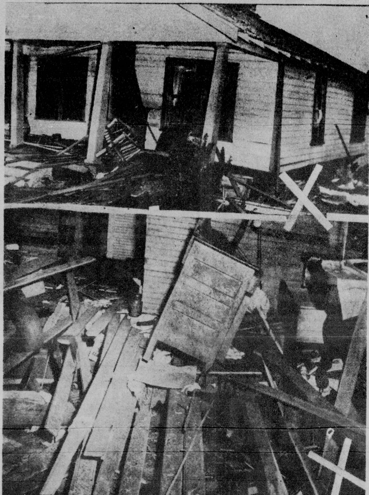
WHERE DEATH STALKED FLORIDA NIGHT—Pictured are interior and exterior views of what was once the modest 6-room home of Harry T. Moore, 46-year-old Florida civil rights leader following a Christmas night bombing in which the former executive secretary of the Florida State branch NAACP was killed and his wife serious-
