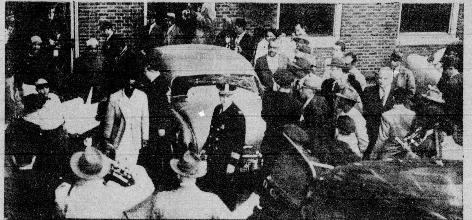
WHERE FOUR LOST LIVES — Hospital and police department workers above remove from a
