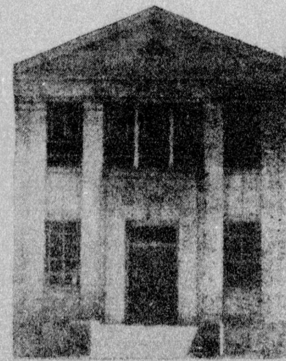
Entrance PENICK HALL Science Building
