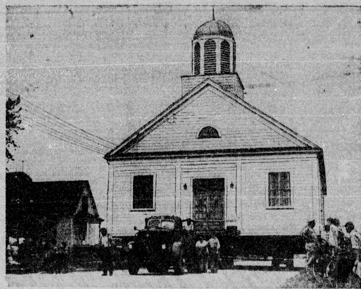
AS GOD MOVES US... The Bethel Reformed church, Phoenix, Ill., is rolling from its former location to a new site in Harvey, Ill. Although the new site is only two blocks from the old, the church must travel in a roundabout circuit, since shorter routes are too narrow for passage.
