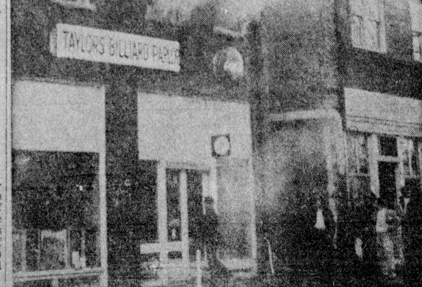
FIRE STRIKES BILLIARD PARLOR APARTMENT HOUSE — A fire, believed to have been caused by an exploding oil stove, completely gutted the inside of Taylor's Billiard Parlor and an apartment house, both located on E. Hargett St., last Wednesday morning. According to occupants of the upstairs dwelling, nothing was salvaged except the clothes that they wore. James Taylor, Jr., owner of the building, had not decided at press time whether he would repair the insured structure. PHOTO BY JONES.
