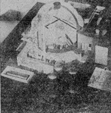
ARMY PACKAGE POWER REACTOR-Model of the Army's auclear power plant. The "package" power reactor is a joint project of the Atomic Energy Commission and the Defense Department. It is the first nuclear plant for providing power and heat for military requirements in remote areas where conventional
