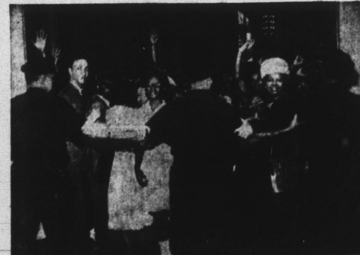
Arms locked, police held back crowd of friends and relatives of 42 integrationists arrested by police last week in Brooklyn, N. Y., when they tried to block construction workers at entrance to the Downstate Medical Center. It was the largest in the wave of Negro demonstrations against alleged discrimination by the city in employment policies.
