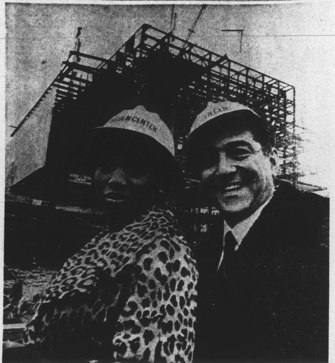
ATTEND "TOPPING OUT" CEREMONY — Soprano Leontyne Price and baritone Robert Merrill of the New York Metropolitan Opera Company attended "topping out" ceremony as the final structural beam is erected at the new house at Lincoln Center for the Performing Arts, there January 20th. The opera company is scheduled to move into the new, $43.7-million house in October, 1966, in New York City. (UPI PHOTO).
