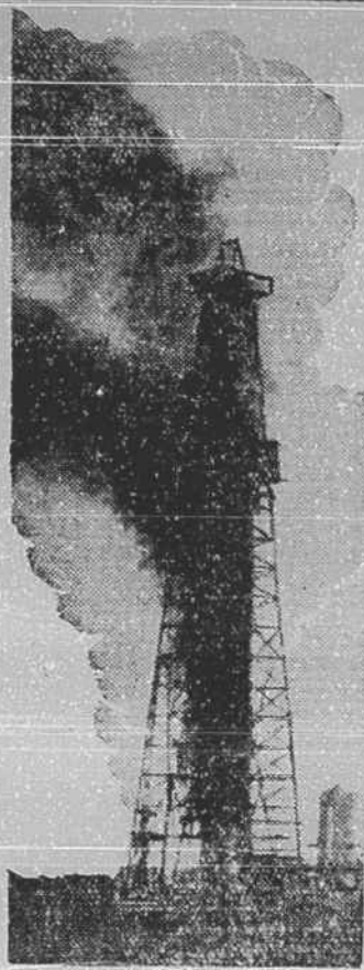
The "Mary Sudik" oil well which threatens the safety of Oklahoma City by the oil spray blown over the town, defies all efforts to cap it.
