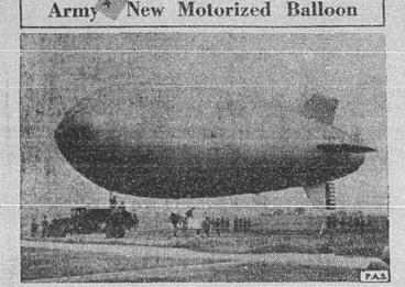
Scott field, Iil.-After six months of experimentation, the war department has decided to construct more of these motorized balloons. They can travel 40 miles an hour under their own power. When anchored to trucks, as shown here, they can be used for observation purposes. The balloons are 100 feet long and cost \$37,000 each.
