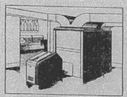
Coal is an ideal automatic fuel to use in conjunction with air-conditioning. Illustrated above is an Iron Fireman DeLaze Hopper model installed in a modern warm air furnace with air-conditioning unit.
