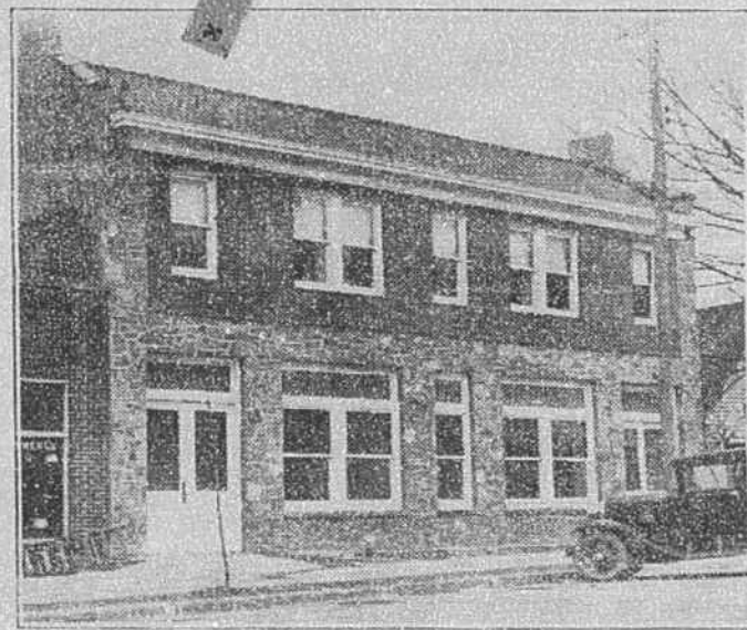
The recently occupied Watauga Democrat building, which is now being used.
