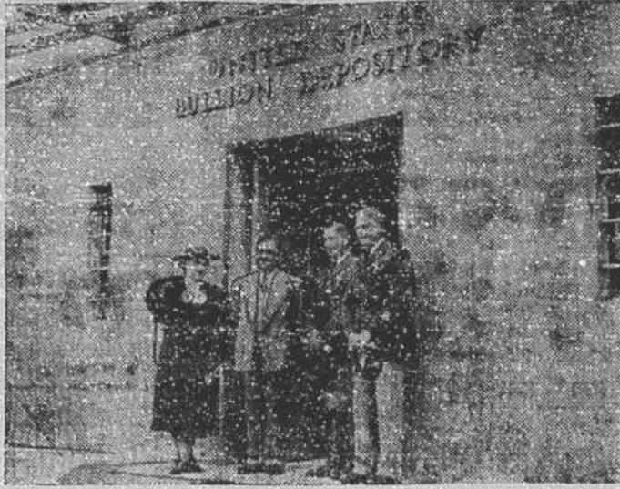
WEST POINT, N. Y. . . . The half-million dollar concrete warehouse the Treasury Department has built on the U. S. Military Academy reservation here will be ready to receive a billion dollars worth of silver for storage on or before July 1st. It has 23 vaults, each large enough to hold 100,000 bars of silver, each weighing 70 to 80 pounds.
