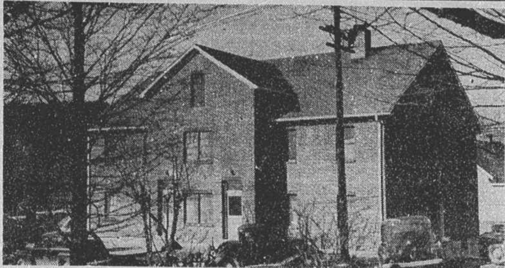
The handsome new medical building recently erected by Dr. H. B. Perry, which is now occupied by Dr. Perry and Dr. R. H. Harmon. The building, which was designed and built solely as a medical structure, can readily be converted into a modern small hospital. The building was occupied early in January.
