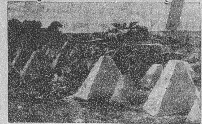
Following a path blasted by U. S. Army engineers, an American tank passes through a belt of concrete and steel dragon's teeth obstacles in the Siegfried line near Aachen.
