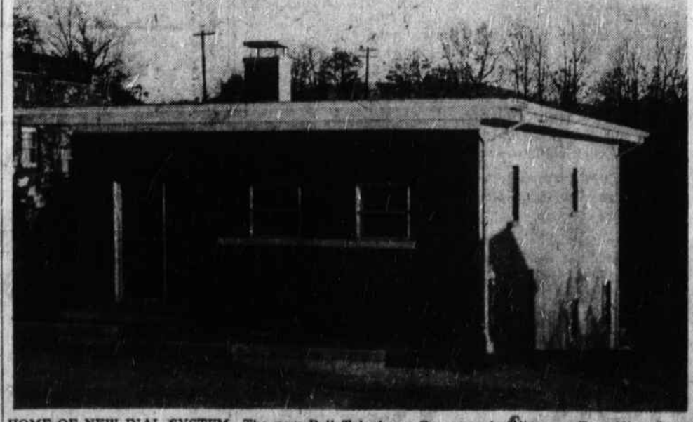
HOME OF NEW DIAL SYSTEM—The new Bell Telephone Company building on East King Street nears completion. Most of the dial telephones are already installed, and the company has announced that it will switch over to the dial system in March.—Staff photo by Joe Minor.
