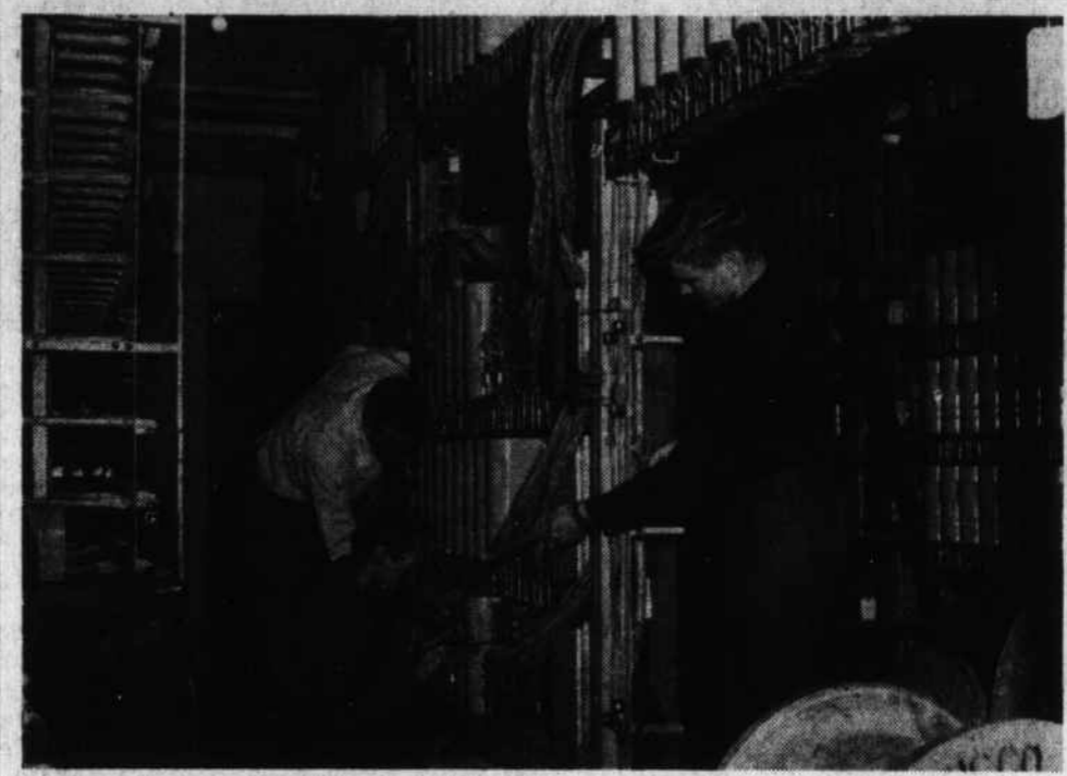
INTRICATE EQUIPMENT—Employees of Western Electric Co. are seen adjusting automatic apparatus at Boone's new dial telephone exchange. They are: J. M. Riddle, G. B. Davis, W. P. Bumpus, J. R. Bryant.—Photo Paul Weston.
