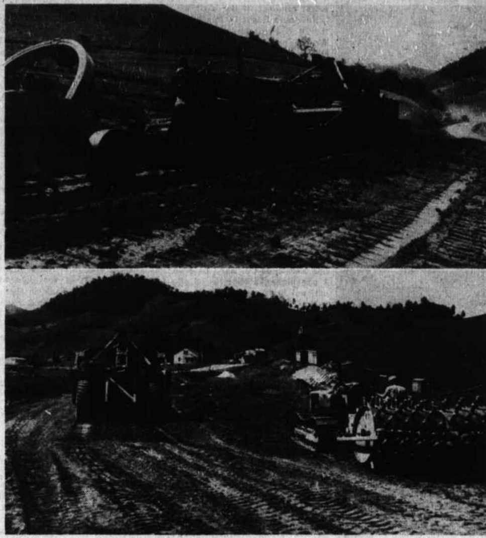
ROUTE 421 STRAIGHTENED—Work on Highway 421, between Vilas and Sugar Grove, is being pushed to an early completion. When the road is finished several dangerous curves will be eliminated on the Ocean to the Great Lakes highway. Shown above in top picture is heavy machinery moving dirt from a 17-foot cut and carrying it to a fill (bottom photo) several hundred yards away where it is being packed and leveled over a culvert.—Staff photos by Joe Minor.
