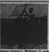
DIAL SUNSHINE-Americus, Ga., farmer George L. Mathews (1) ma the historic first call over a telephone using power from Bell Labora-tories' amazing new sunshine battery. One of the new units, which con-verts light into electric current, is shown receiving final adjustments by Southern Bell cable repairman B. W. Kennon.
