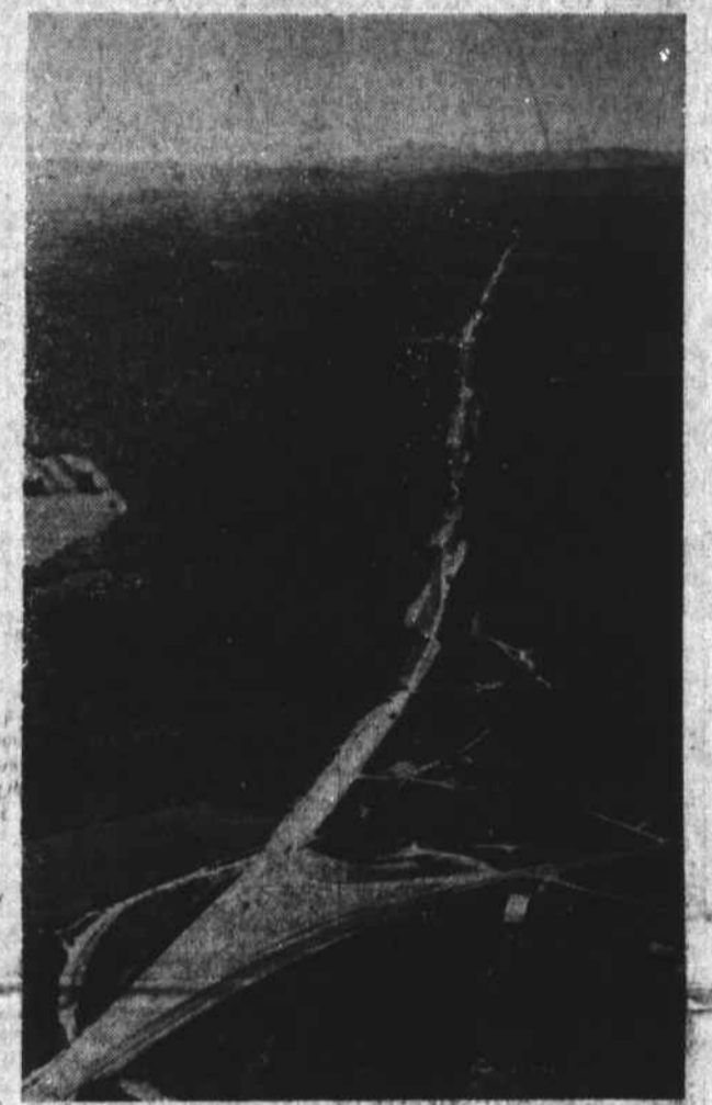
The roadbed of the new 12-mile stretch of U. S. 421 takes almost a straight line through the mountains between Wilkesboro and Boone. Two million cubic yards of earth were moved in straightening this main east-west artery. This view looks west from the edge of Wilkesboro toward Grandfather Mountain, 37 air miles away.—Photo by Max Tharpe, courtesy Highway Commission.
