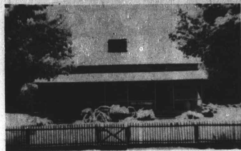
THE OLDEST LOG HOUSE . . . Built around 1780, the log house owned by Mr. and Mrs. Charles Wilkinson of Zionville is no doubt the oldest structure of its kind in the county. The logs from which the house is built were hand-hewn with a broad axe, and there's a double chimney built of rocks, with five-foot fireplaces in each end. The main structure consists of four rooms, each 17x18 feet, with two rooms up and two down, with an outside stairway. Additional rooms have been added four different times. More than 20 different families are known to have inhabited the house, Mrs. Wilkinson says, but it has remained in the hands of some member of the original family down through the years.
