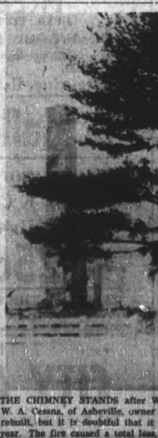
THE CHIMNEY STANDS after Watauga Inn at Blowing Rock was destroyed by fire early this month. W. A. Cessna, of Asheville, owner of the popular resort hotel, stated this week that the inn will be rebuilt, but it is doubtful that it will be ready for use this summer. It probably will be opened next year. The fire caused a total loss, according to fire men.—Photo by Palmer's Photo Shop.
