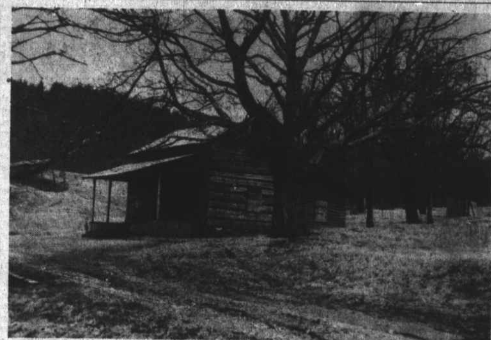
BOONE LANDMARK . . . The Thomas Greer House, one of the oldest structures in the town, is said to have been built between 1865 and 1868. Mr. Greer, who moved from the head of Elk after the marriage of his daughter to T. J. Coffey, died there. It is built of hewn logs, fashioned largely by Cap-
