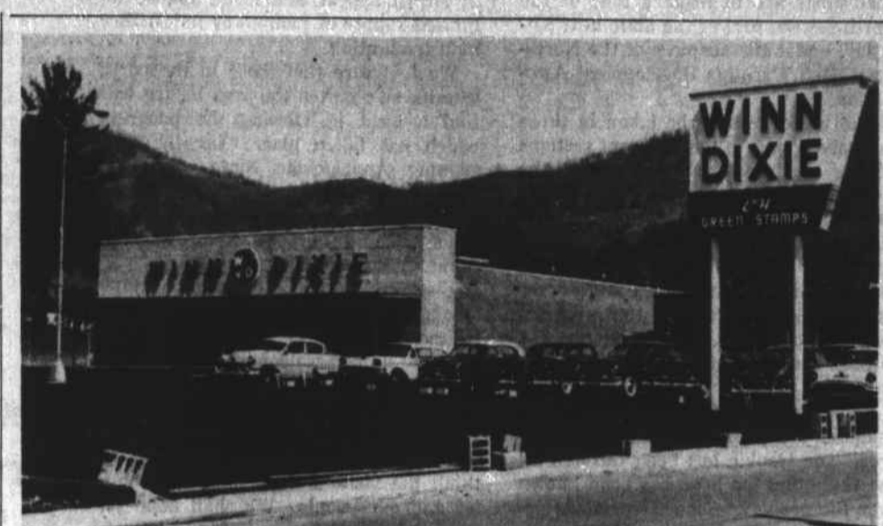
NEWEST STORE.—The finishing touches were just being completed on Winn-Dixie's newest store on Hardin Street and Blowing Rock Road, as this photograph was taken. Part of the large, hard-surfaced parking area is also shown. This is Winn-Dixie's newest store.
