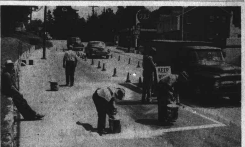
TRAFFIC IMPROVEMENT. —State Highway sign crew paints arrows and stop lines at spot light on corner of East King and Hardin streets. The arrows direct traffic into right-turn-through lane and left-turn lane, designed to cause smoother flow of traffic. As one of the workmen said: “It ought to help—if it works!” Judging from driver comment, it does work. Left-turn traffic now stops several feet back of through traffic, to allow easy passage of trucks and other vehicles making a right turn off Hardin street.—Staff photo Joe Minor.
